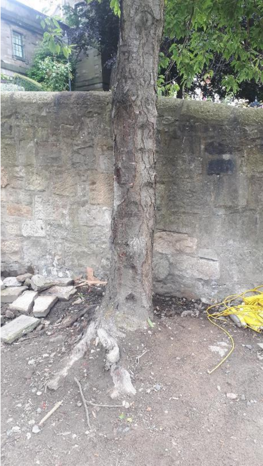
Figure 3 The image supplied by the agent showing ground disturbance and compaction
